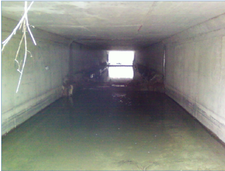
Site 2 Beitz Drain at Six Mile looking upstream
