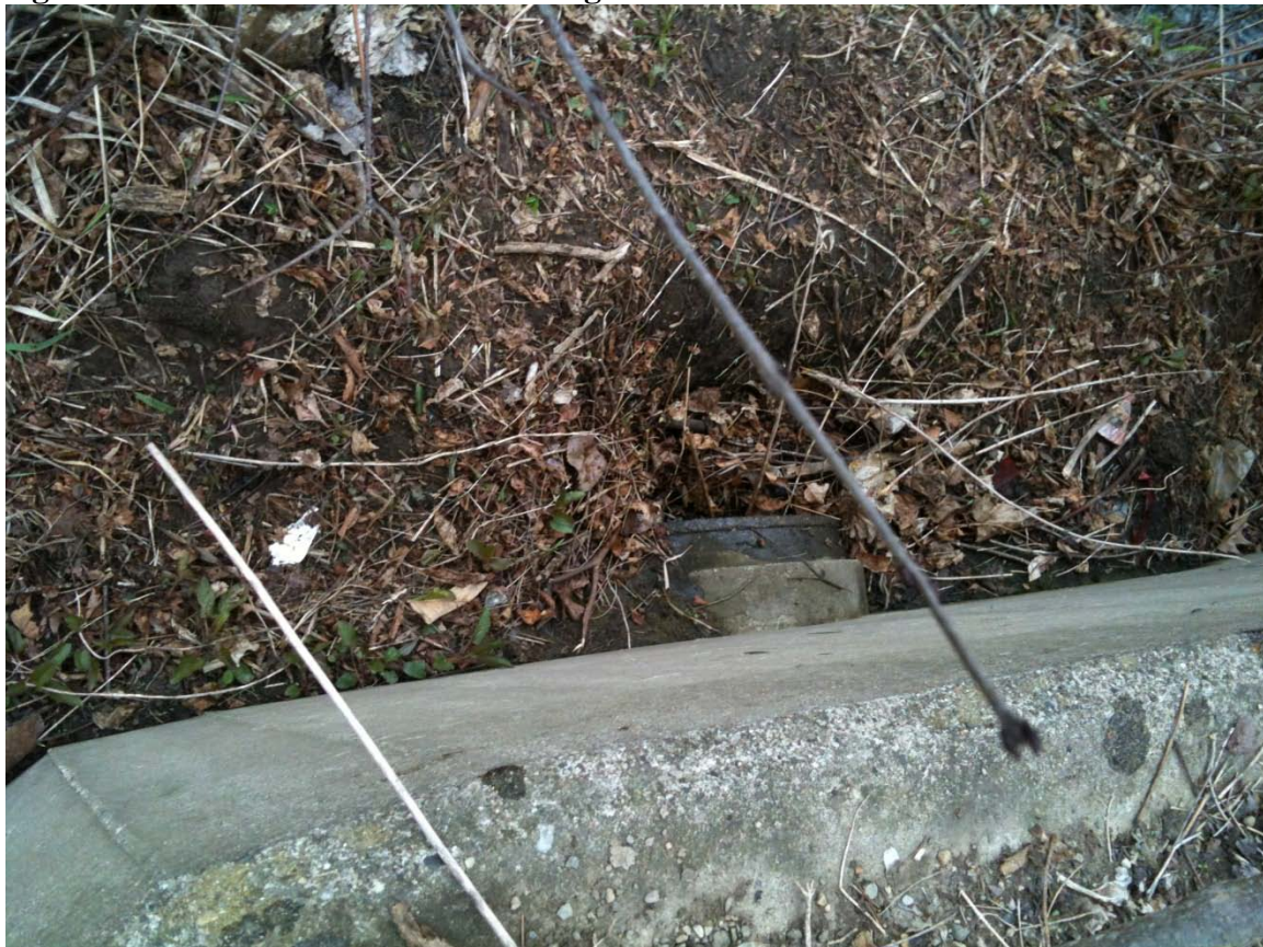
Figure 4: Private Storm Sewer Discharge to the Johnson Creek
