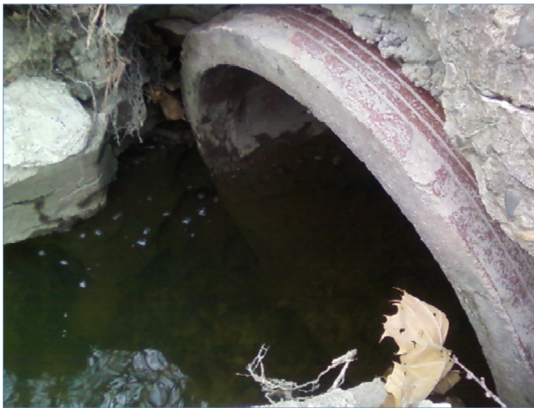
Site 3 Park Street Outfall
